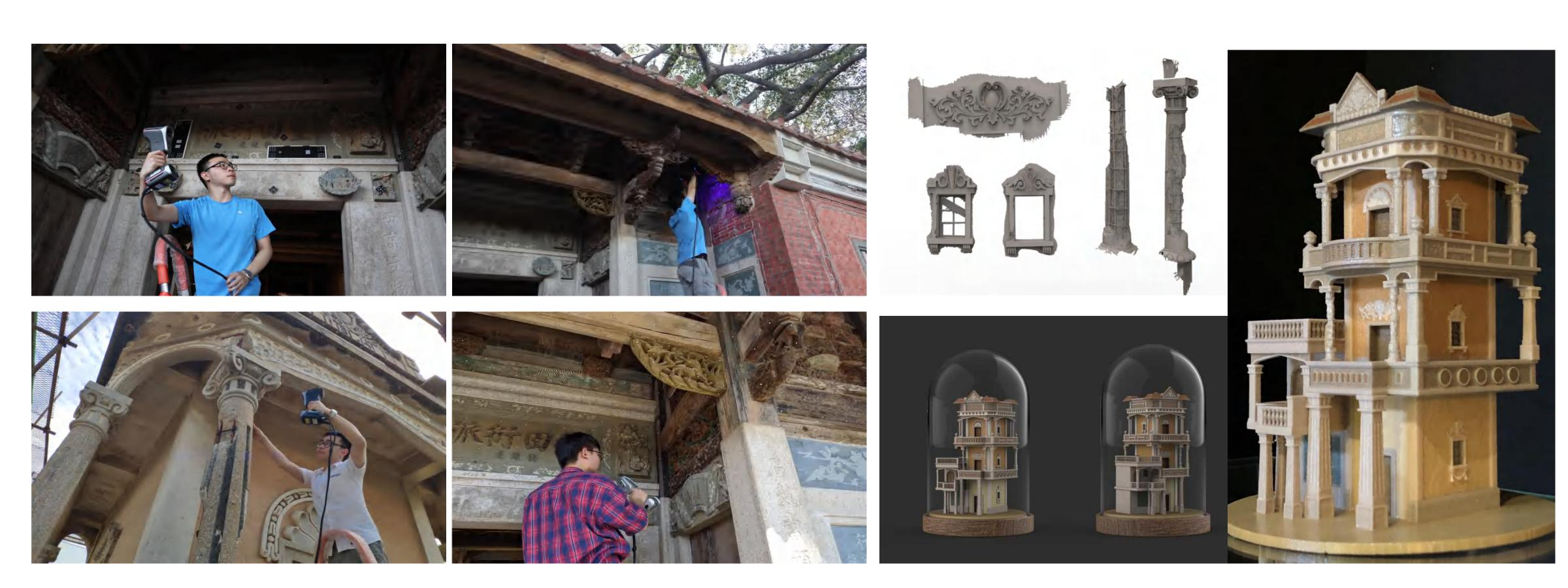
Field study → Partial scanning of buildings → Data processing (forward + reverse) → 3D printing
